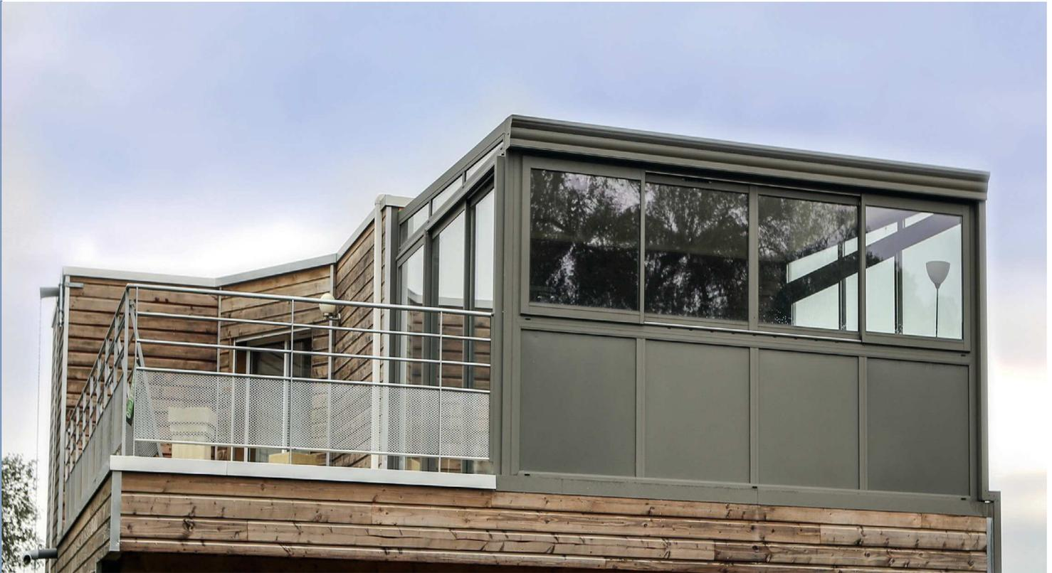
The **double-sided technobond panels** are part of the **CONSERVATORY** product range. They are assembled with a self-adhesive hot-melt film based on an extruded polystyrene rubber.
